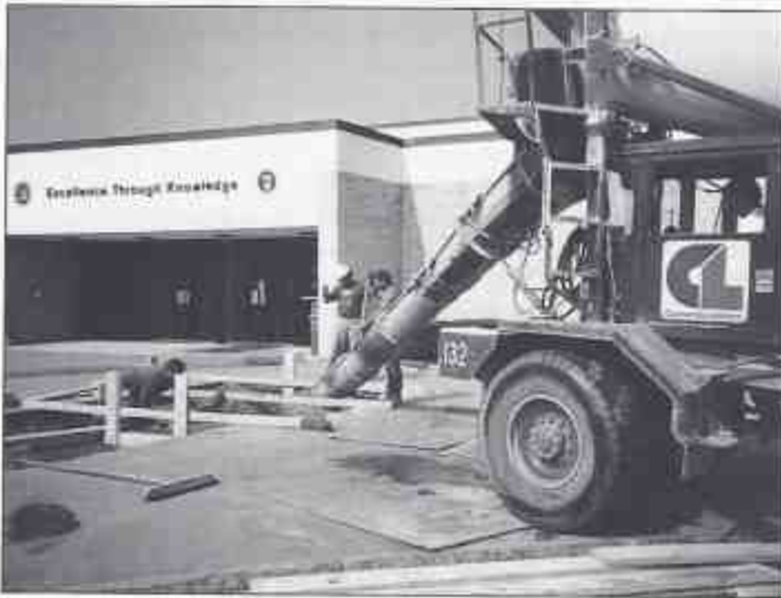
Clemente-Latham Concrete Corp. pours the footing for monument and base.
